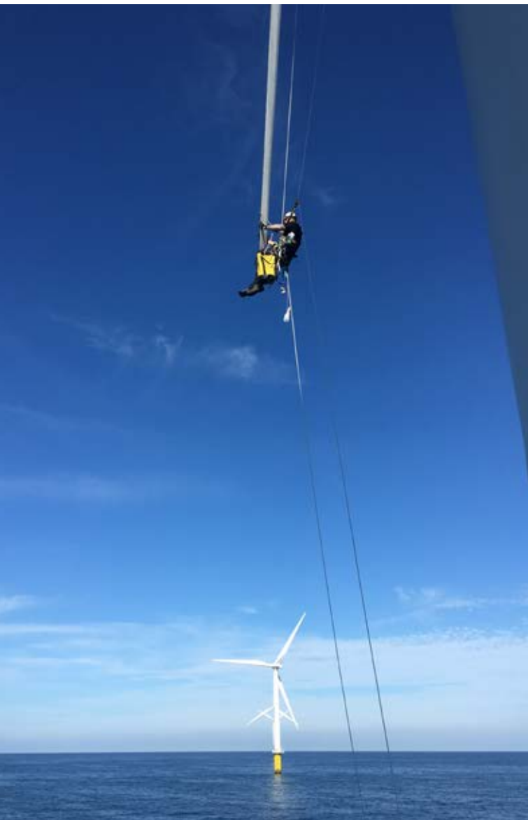
Servicing work at an offshore wind farm
