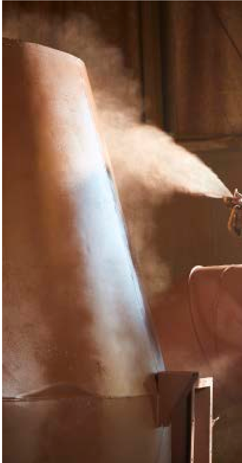
Application of corrosion protection
