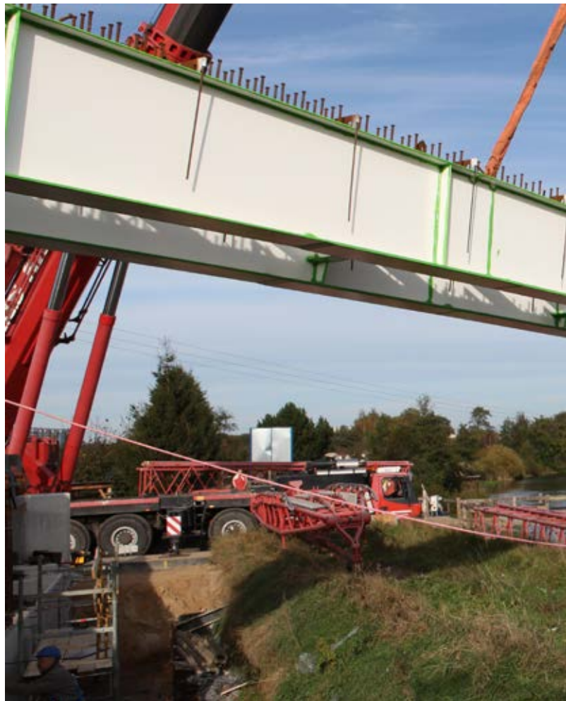
Construction of a steel bridge
