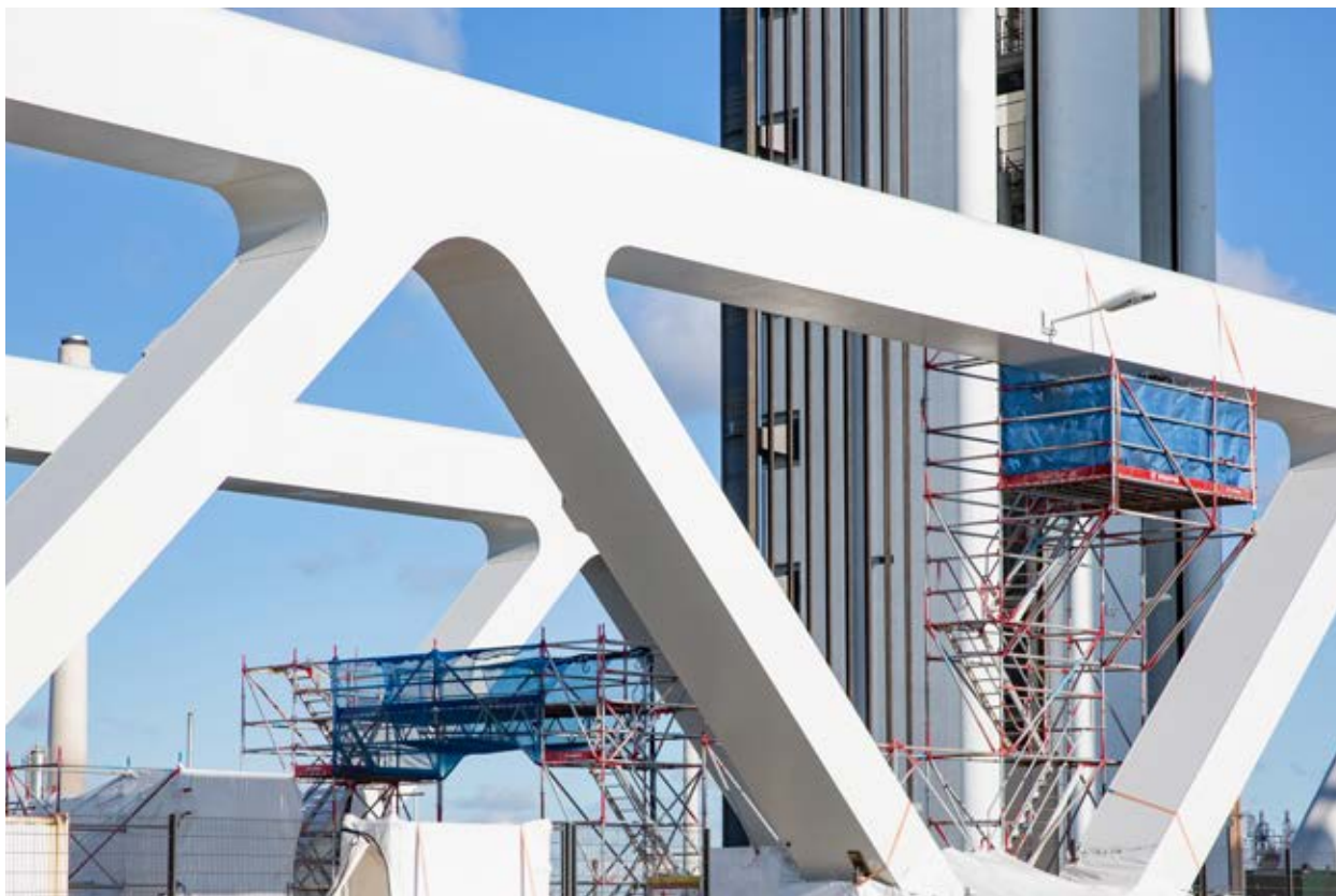
Application of surface protection
