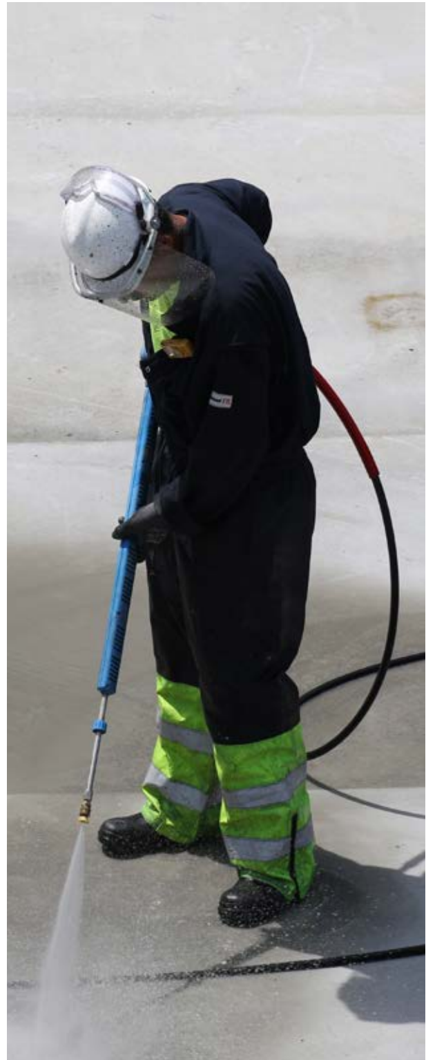
Preparation for corrosion protection work
