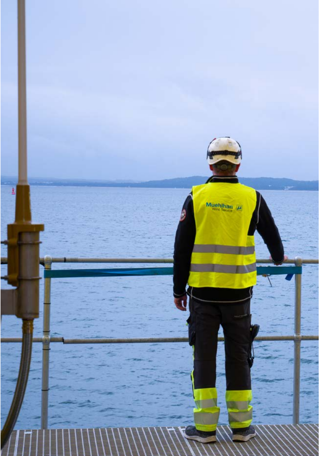
Servicing work on an offshore wind turbine
