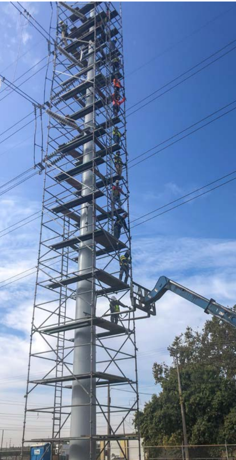
Specialty access and scaffolding
