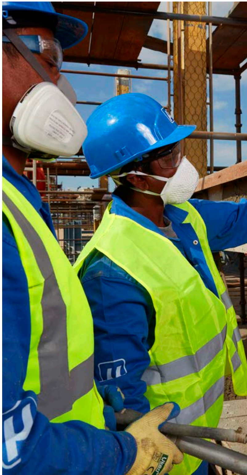
Application of passive fire protection
