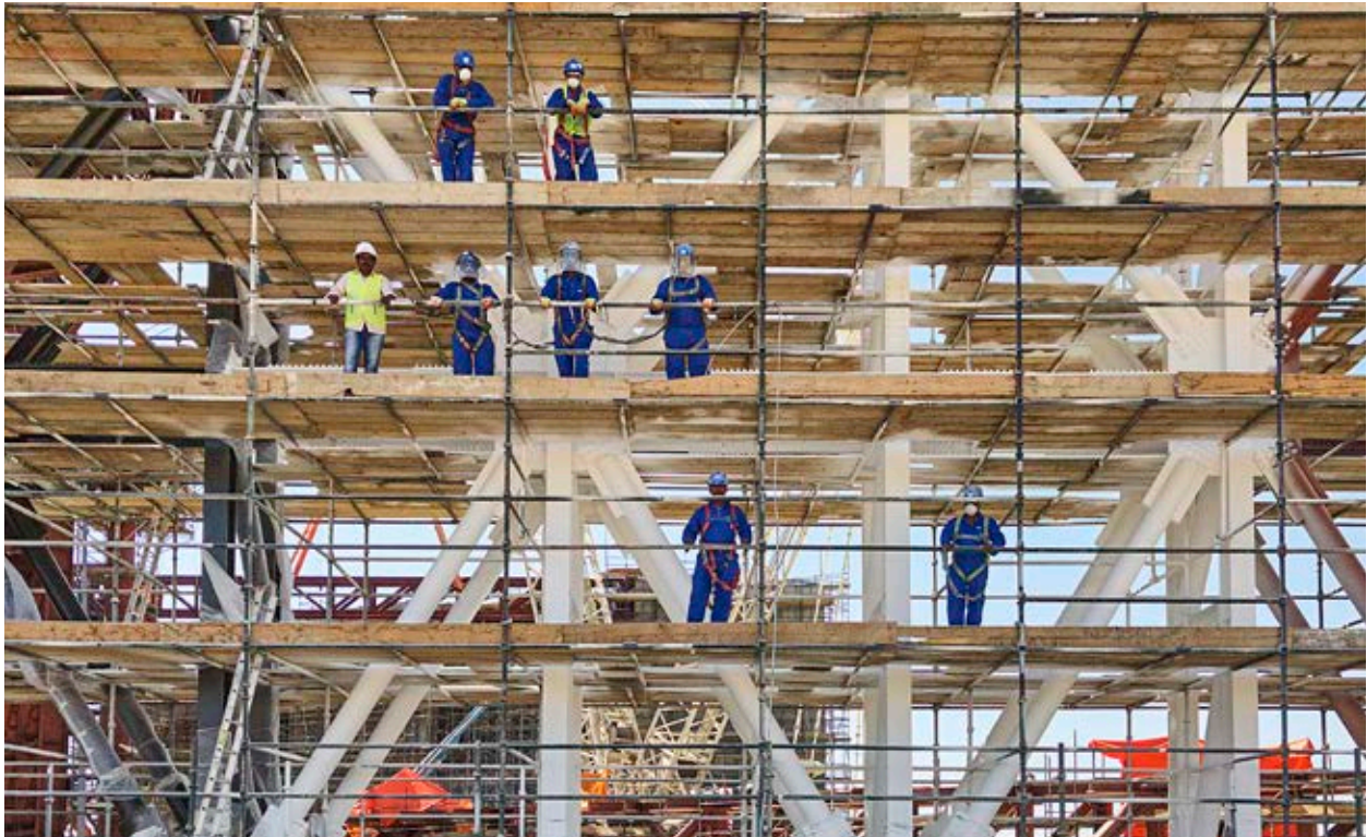
Fire protection work at the Across Ages Museum, Nizwa, Oman
