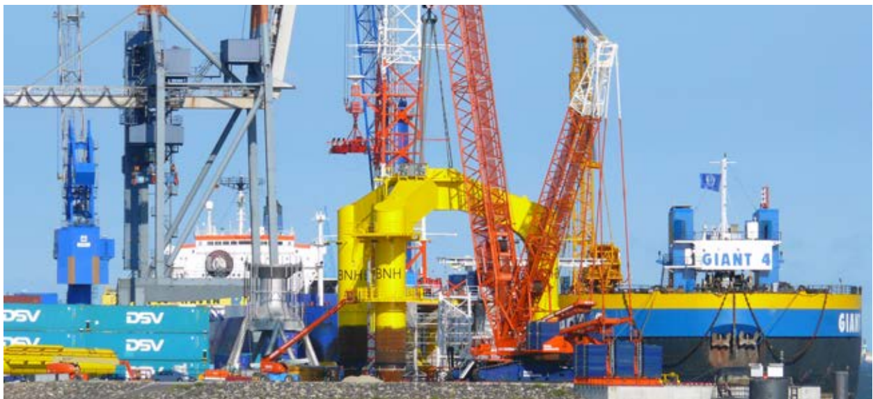
Loading of tripods for an offshore wind farm in Hooksiel
