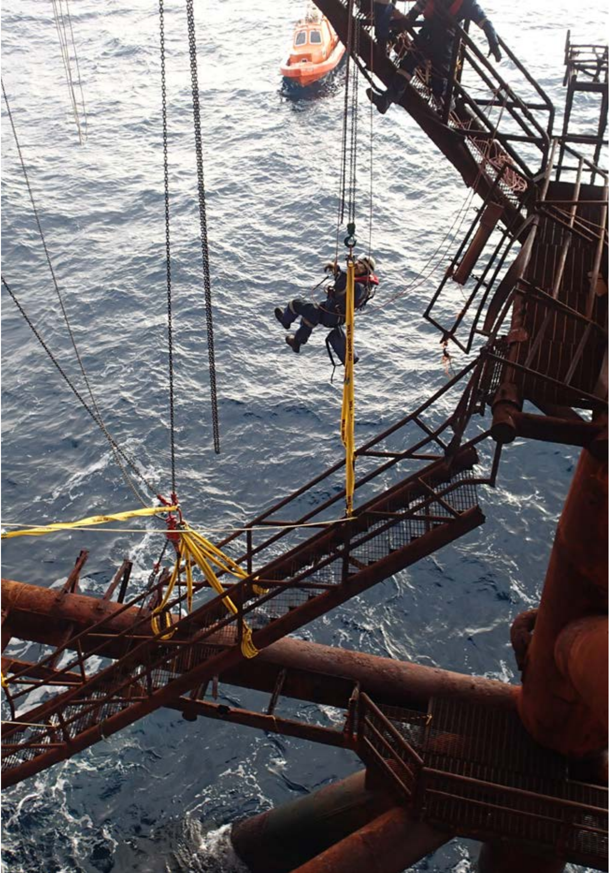
Access technology on an oil platform
