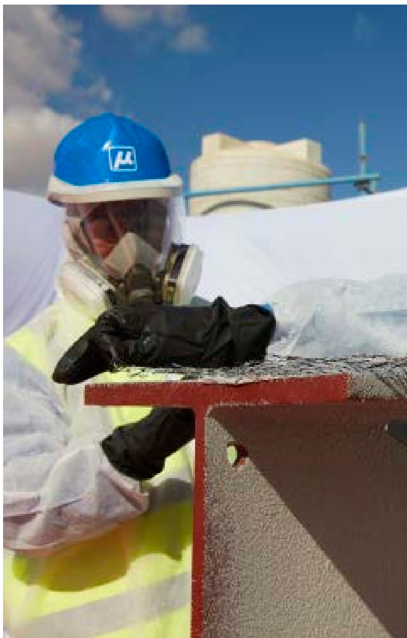
Application of passive fire protection
