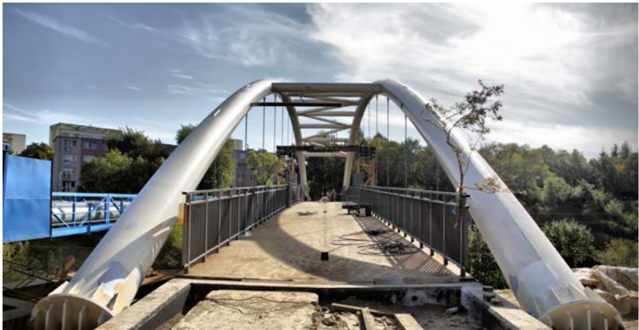
Construction of a steel bridge
